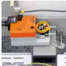
Automatic air supply and exhaust air flaps
