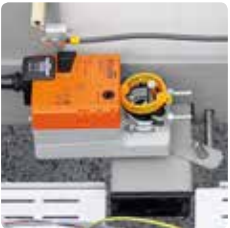
Automatic air supply and exhaust air flaps
