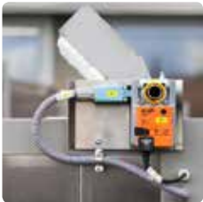
Automatic exhaust air flaps
