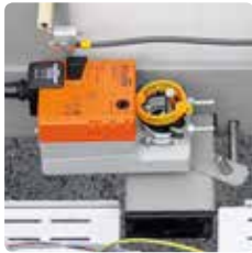
Automatic air supply and exhaust air flaps
