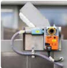
Automatic exhaust air flaps
