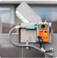
Automatic exhaust air flaps
