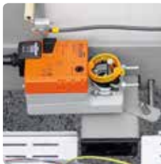
Automatic air supply and exhaust air flaps
